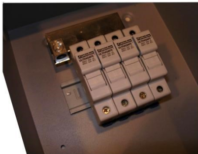
4 Touch safe fuseholders installed in an MNPV6
